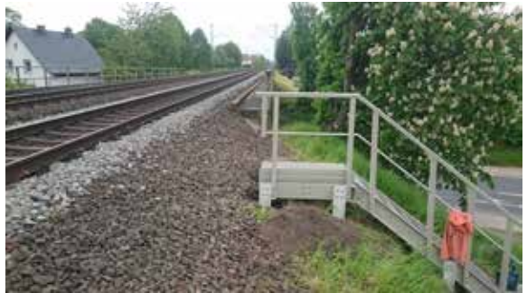
Embankment stairs, Friedberg
