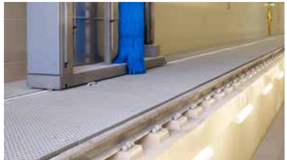
Keolis washing bay, Hamm
