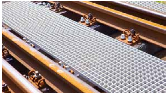
Bridge over the Main, Haßloch
