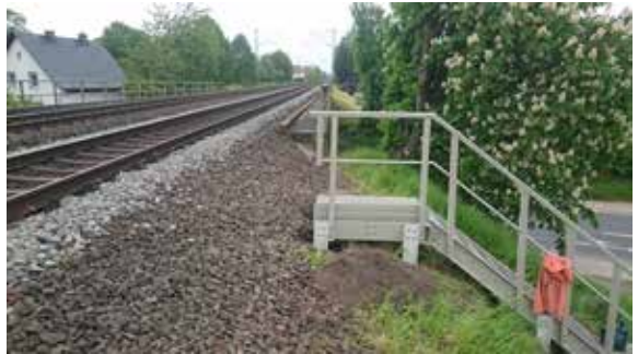
Embankment stairs, Friedberg
