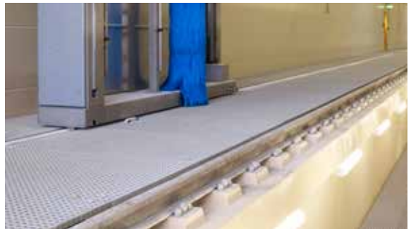
Keolis washing bay, Hamm
