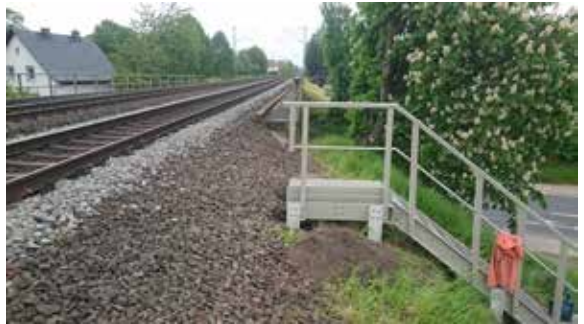
Embankment stairs, Friedberg
