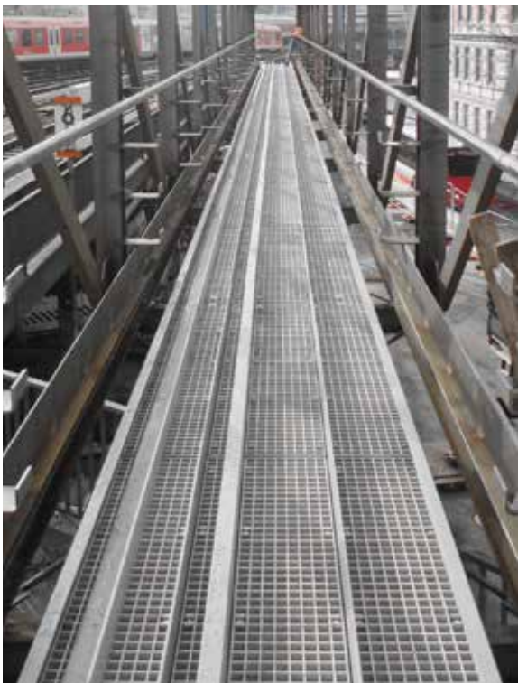
both pictures Cable bridge EÜ, Hamburg
