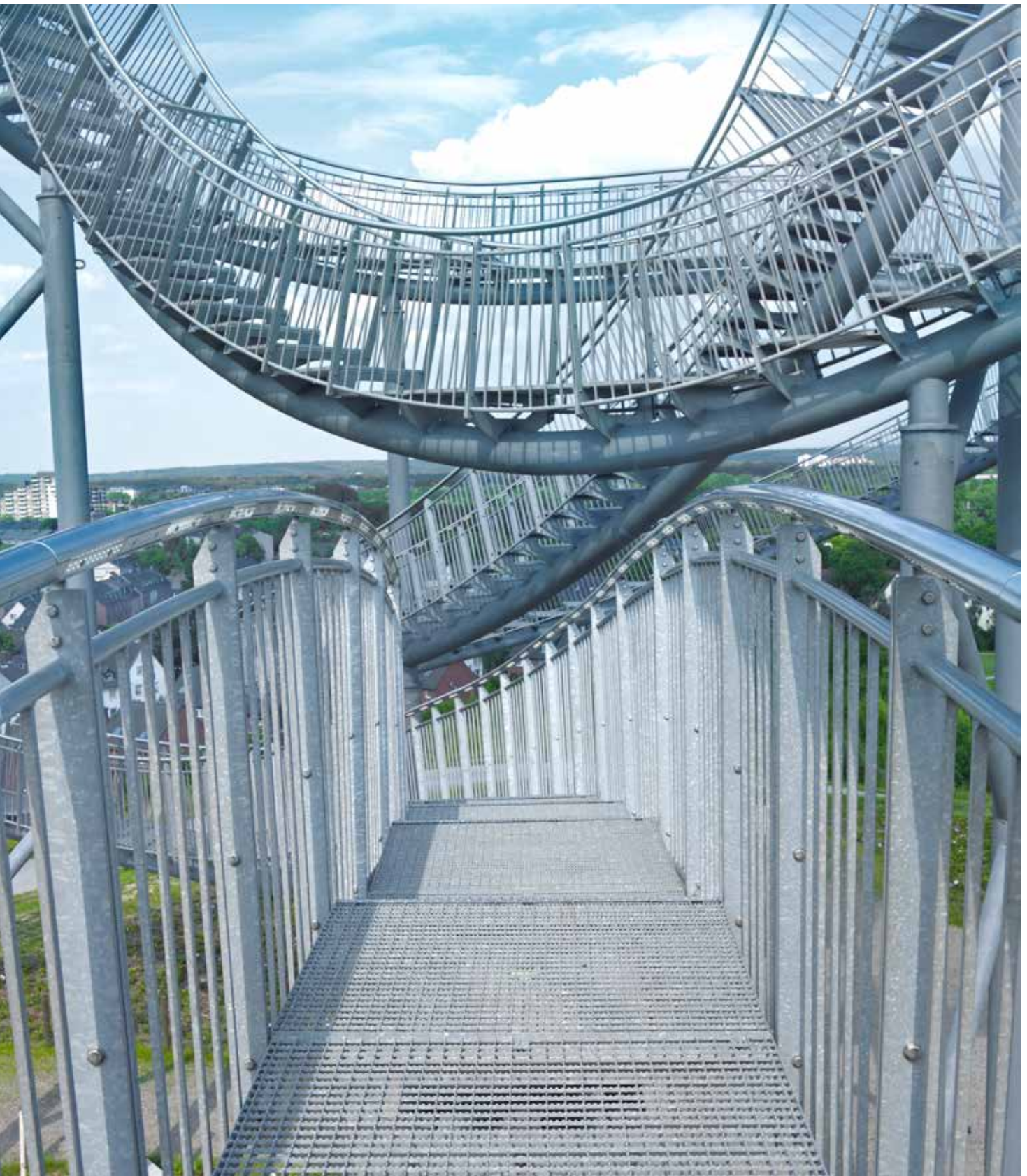
On the walkable roller coaster Tiger & Turtle, MEISER press gratings with anti-slip protection provide secure footing at lofty heights
