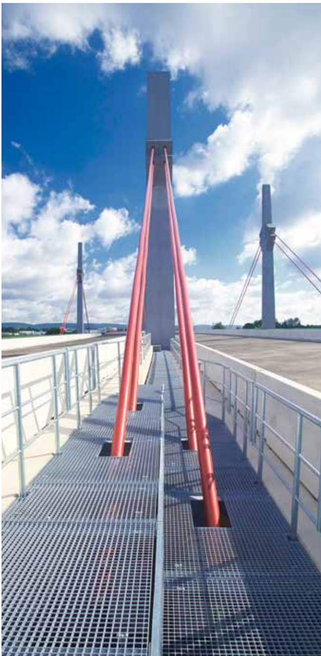
MEISER gratings used as a walkway on the Bad Oeynhausen bridge
