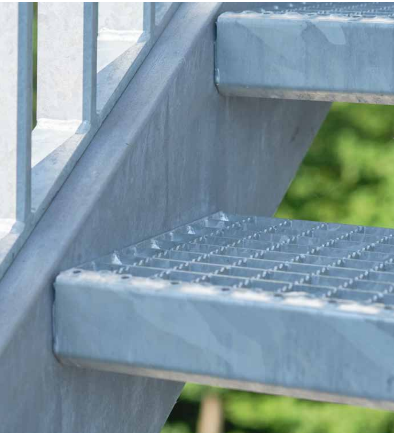
Perforated metal steps with anti-slip surfaces at the Gobelwarte Grein
