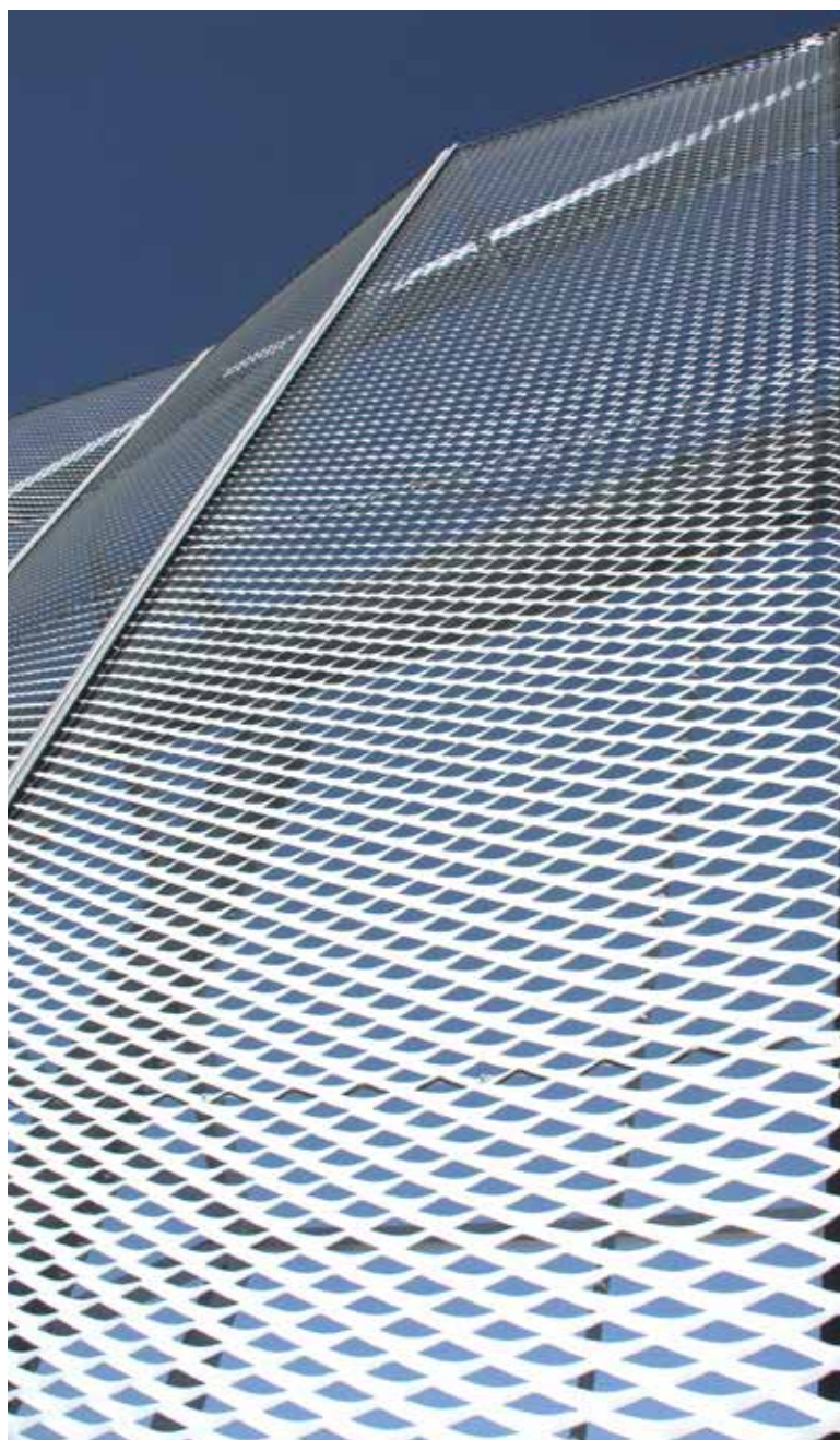
On the façade of the Bilbao Exhibition Centre in Spain, MEISER expanded metal gives the architecture a modern and distinctive appearance
