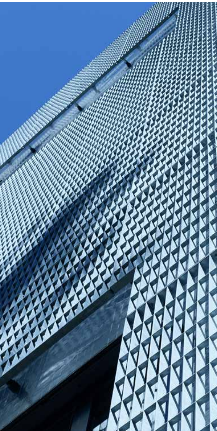
The façade of the École St. Sophie, clad with MEISER press-formed gratings
