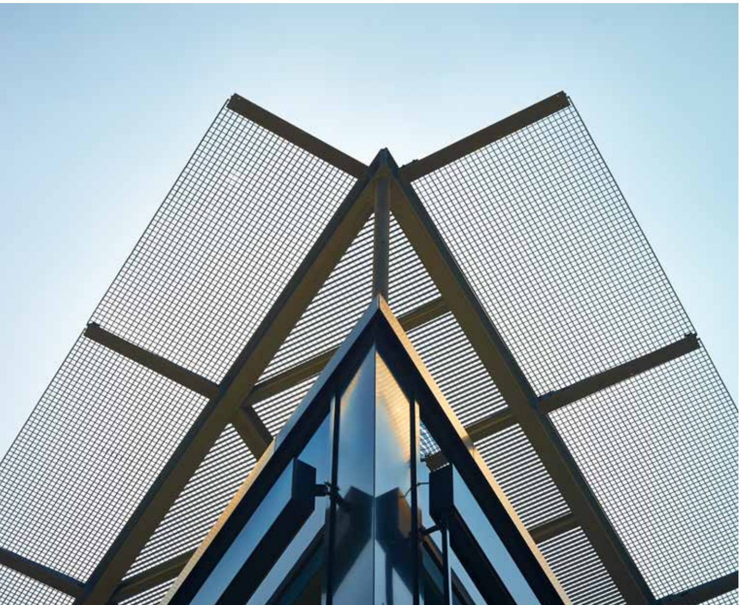
Gratings used for shading in Freiburg-Hochdorf
