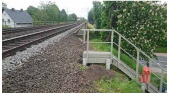
Embankment stairs, Friedberg
