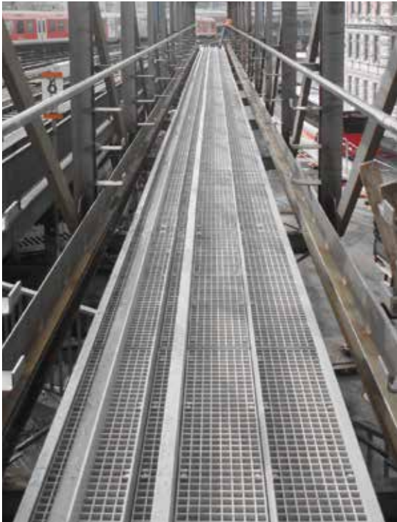
both pictures Cable bridge EÜ, Hamburg
